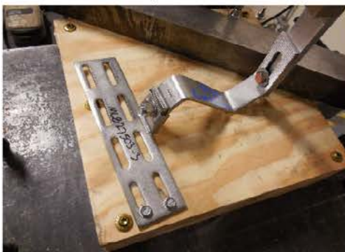
Photo 7: Hook Contact with Plywood
